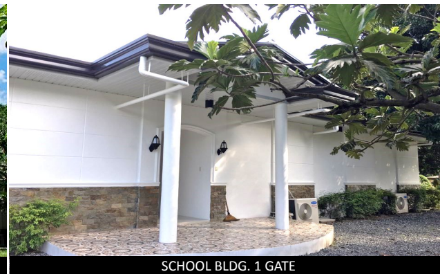
SCHOOL BLDG. 1 GATE
